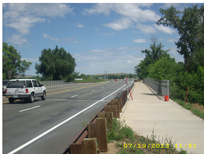
SV-13A LOOKING NORTH
